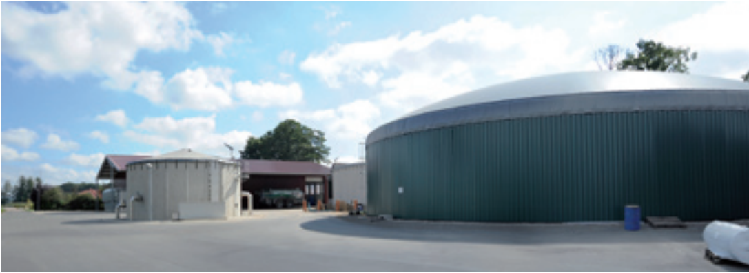
The biogas plant has been providing heat for the own agricultural business since the end of 2007
