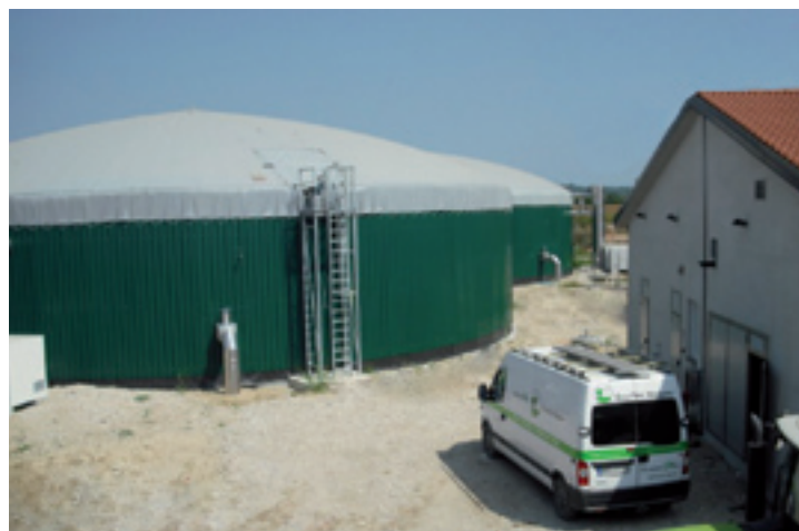
Biogas plant in Volta Mantovana
